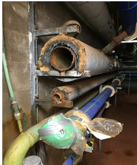
*Aquatherm blue pipe system replaced the corroded black steel pipe systems.*
