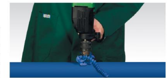
Drilling through the pipe wall
