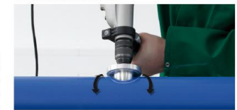
Removal of the oxygen barrier layer
