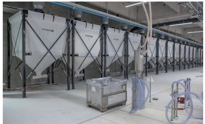
Upstairs the periphery for pipe material supply is formed
