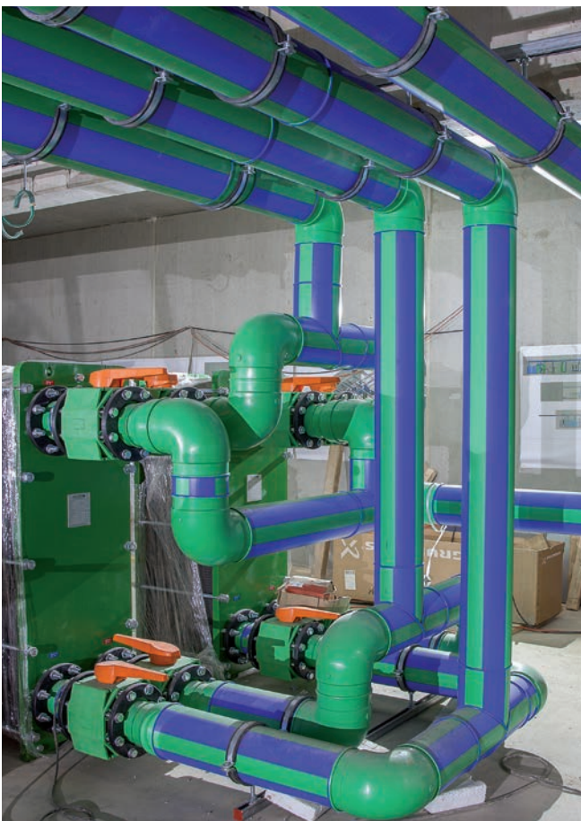
Commissioning of the system for process cooling
