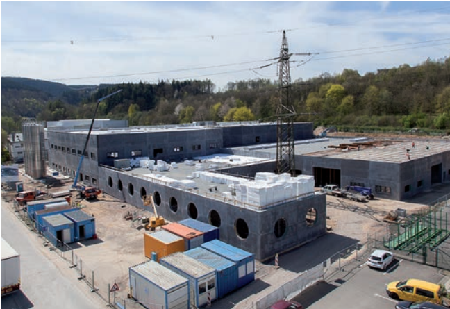
View from the technical office
