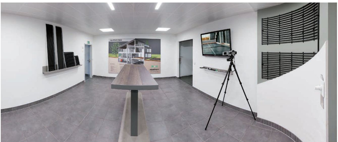
Room 2 demonstrates a single-color metal panel ceiling. Here the aquatherm black system is integrated as a square and rectangular panel with different lighting. Even the application in curves is impressively presented. An infrared camera visualizes the function of the heating and cooling panels for the visitors.
